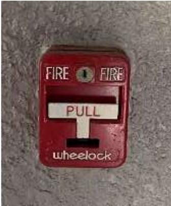
**Fire Alarm Pull Station:** The fire alarm pull stations are located on each end of the building at the stairways. To activate simply PULL the white handle. Remember to call **9-1-1** after activating a fire pull station.
