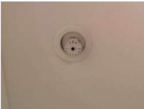
**Sprinkler Activation:** Smoke **DOES NOT** activate a sprinkler head. The sprinkler heads are activated by heat generated by fire. If the sprinkler head is activated by fire or other damage, the fire alarm monitoring service will notify the fire department.
