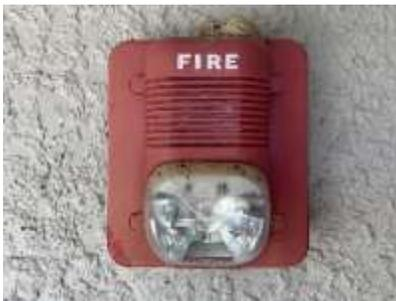
**Building Fire Alarms:** The building fire alarms are located on the exterior wall on each floor level. The building fire alarms will emit a high-pitched sound and a strobing white light. When the building fire alarm is activated, immediately exit your unit and use the stairways at either end of the building to the ground floor. **DO NOT** block the elevator lobby.
