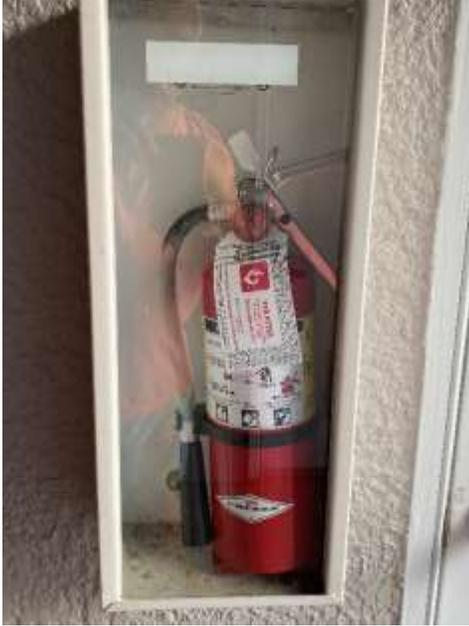
**Fire Extinguishers:** There are fire extinguishers located on each floor at various locations. All of the fire extinguishers are **A B C**. The “A” indicates use on ordinary combustibles, wood, paper, cloth, etc. The “B” indicates flammable liquids, grease, oil, paint, solvents. The “C” indicates use on live electrical equipment, electrical panel, electric motor and electric wiring.
